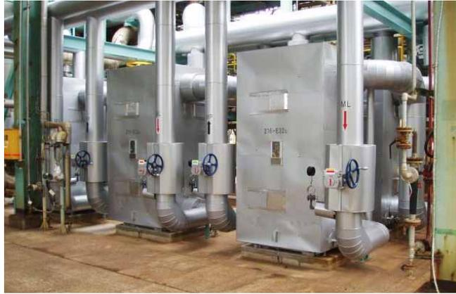
Exchanging their existing coil-wound heat exchanger for four Alfa Laval Compablocs eliminated the severe fouling problems the plant struggled with before.
