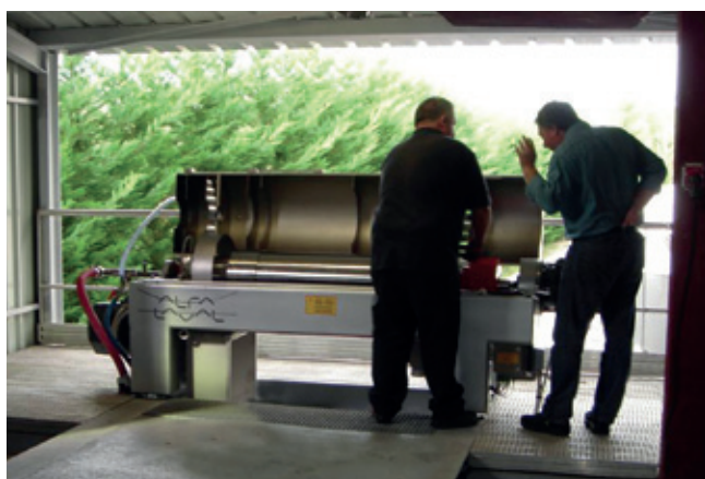
Installation of the Foodec decanter at Rabastens
