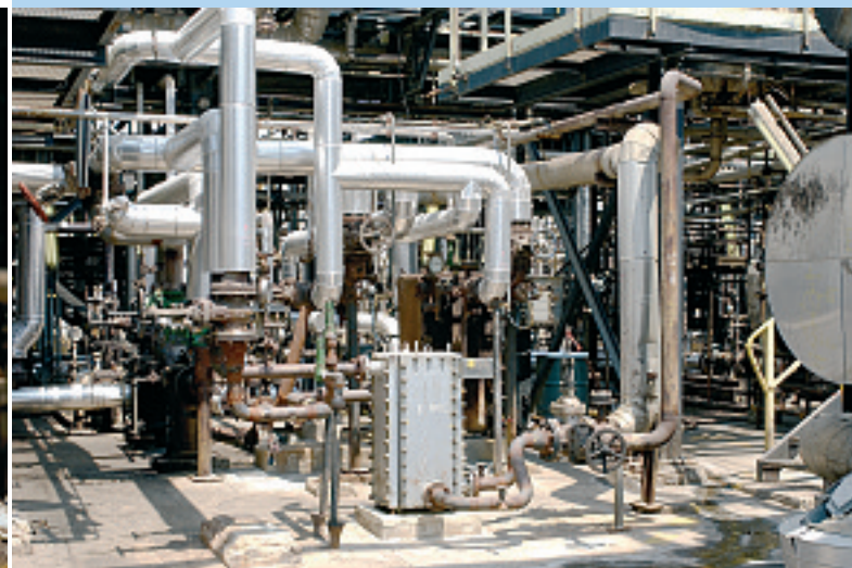
The Compabloc heat exchanger in the SWS plant is perfect for handling high temperature fluids.
